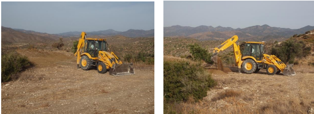
Figure 6.1.5: A JCB mechanical digger excavated a trench at the site of Parsata borehole 3 (see appendix 1). The full trench log is presented in appendix 2.
