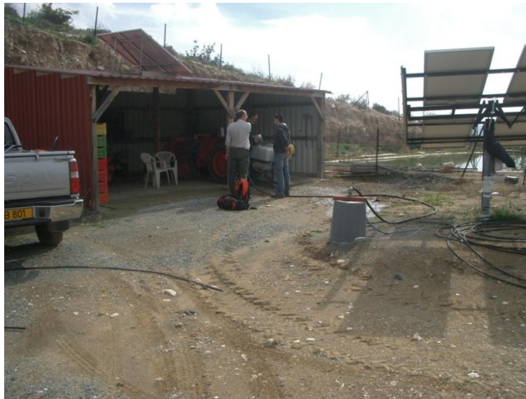
Figure 5.1.3: Typical pumped well (grey cylinder in middle ground) at the Almond Orchard near Parsata, southwest Cyprus (looking south). Note the government-issue solar panels which power the pump are generally a good indicator of the presence of a borehole.
